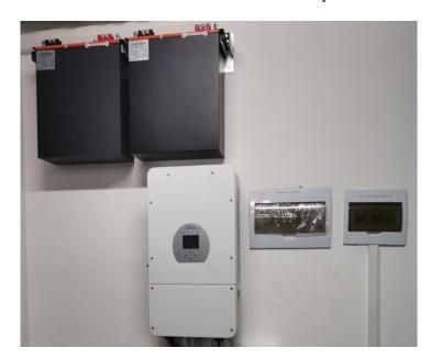
The system is designed to optimally produce Solar Power to supply continuous power to essential loads in the building and charge the battery. The AC Electrical works will be custom designed to meet the essential load backup requirements during load shedding. The batteries will charge and discharge (Cycle) stored power each day to optimize the performance of the Solar system. Should the batteries be full and there are only small loads the PV production will be throttled unless power is exported
